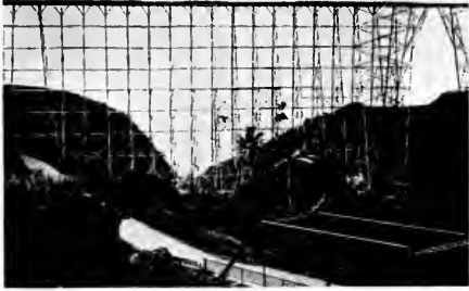
High trestle carrying water flume, a frequent sight in the Hawaiian Islands.
